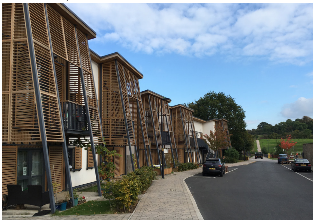
Fig. 51 | Exemplar sustainable buildings, Hanham Hall, Bristol
