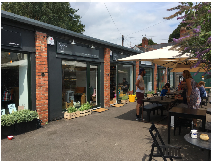
Fig. 54 | Retail units in light-weight, temporary structures with active outside spaces, Cardiff
